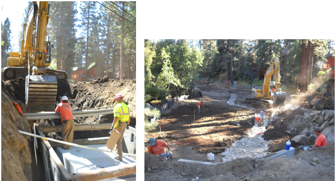
Figure 10. Left: Installation of the culvert presented difficulties as many existing utilities were present. Right: The construction of the channel immediately downstream of the newly installed culvert.
