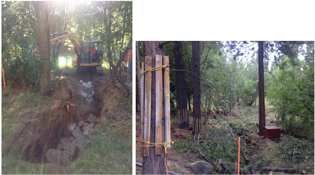
Figure 14. Left: With the water diverted from the old creek location to a pipe for the construction of Phase III, the monitoring station had to be moved upstream of Northwood. Right: The portion of the valley-wide grade controls that crossed the existing channel had to be constructed during Phase I and marked with a 2x4 so that the Phase III portions could be aligned.
