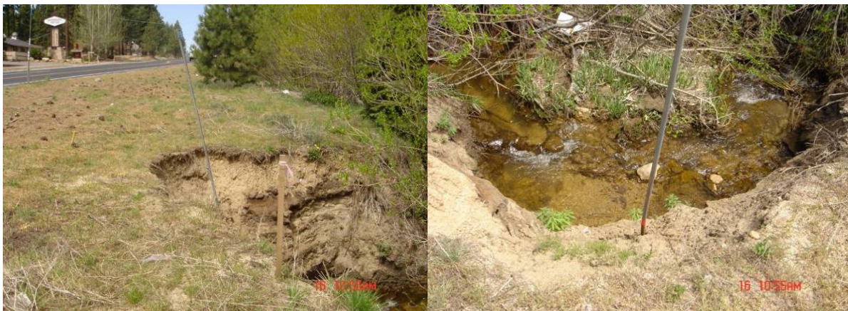
Figure 4. Photos of the large headcut near the crossing at State Route 28.
