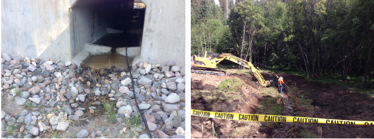
Figure 13. Left: Construction of the upstream tie-in. With the completion of this tie-in, the new Rosewood Creek channel could finally receive flow. Right: The new Rosewood Creek culvert receiving flow for the first time on September 11, 2014.
