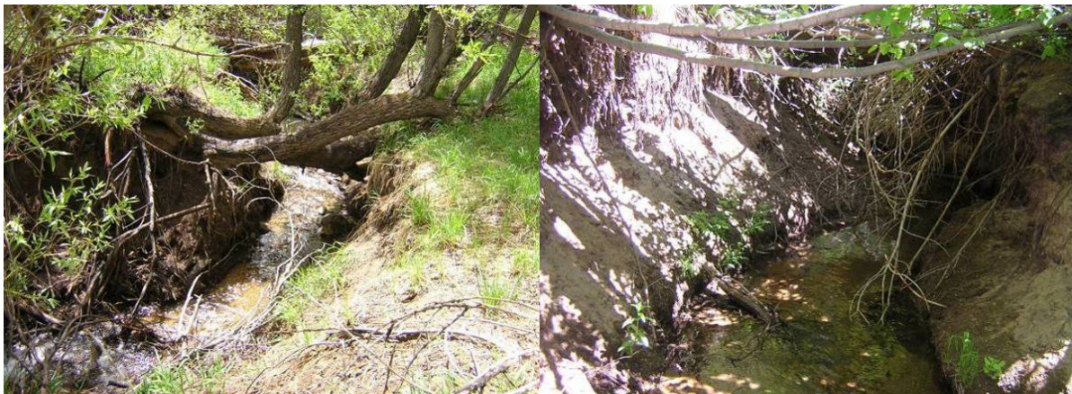
Figure 6. Photos of the large headcut near the crossing at Northwood Blvd.
