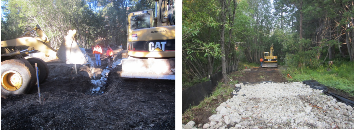
Figure 9. Left: At the beginning of Phase I, an access road was built into the project area and numerous willows and alders were removed. Right: The construction of valley and channel wide grade control structures involved placing subsurface rock.
