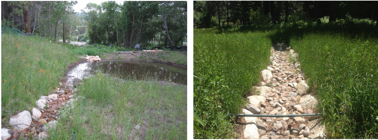
Figure 11. Left: Phase II, June 2013, vegetation showing remarkable success. Right: Phase II, July 2013, having an area at the bottom of the inactive channel for water to pond was essential for erosion prevention.
