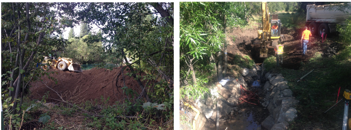
Figure 12. Left: Construction of the downstream tie-in occurred at the beginning of Phase III. Right: Filling the old channel commenced after the construction of the downstream tie-in.
